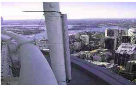
*Flat Panel Antenna Mounted at Receive Site*
